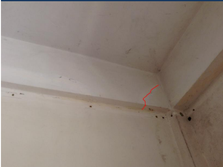
Cracking in beams
