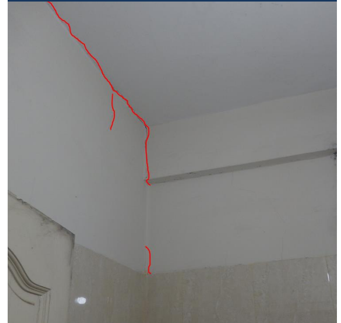
Cracking in walls
