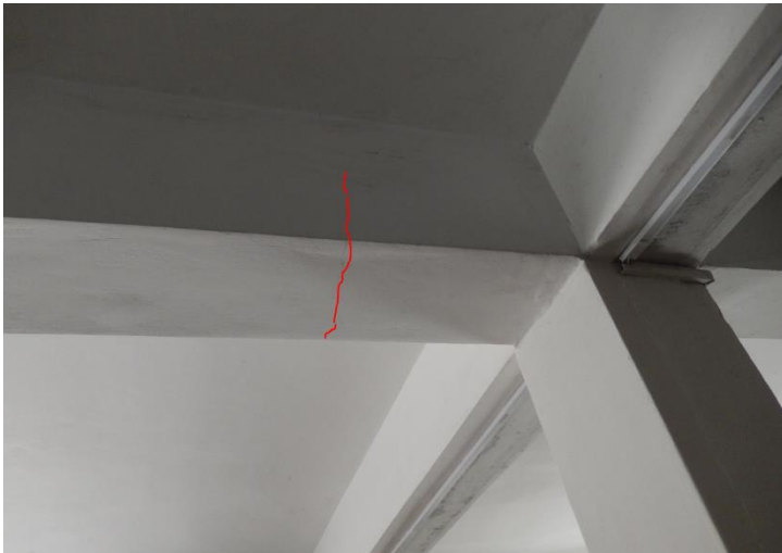
Cracking in beams
