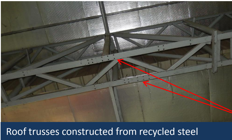
L-purlins appear not adequate to resist high wind loads
