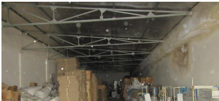
Internal wall with cantilevered cavity beam for rain water drainage
