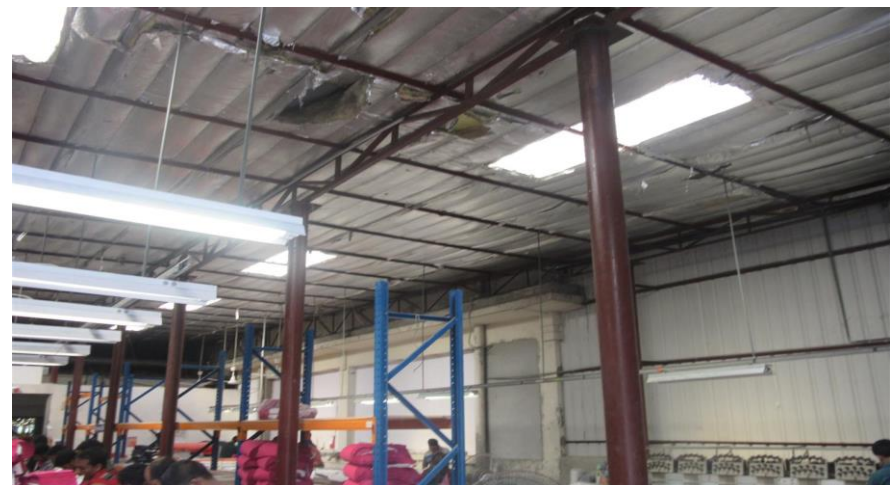
1 Storey Steel structure
