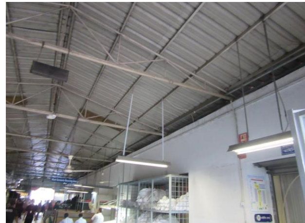
4. – Infill between B2 and adjacent building
