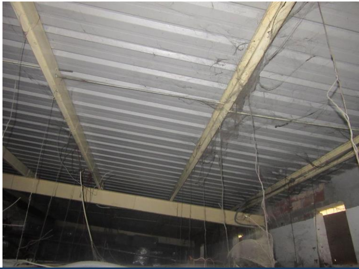
1. – Northern Extension of Building 1
