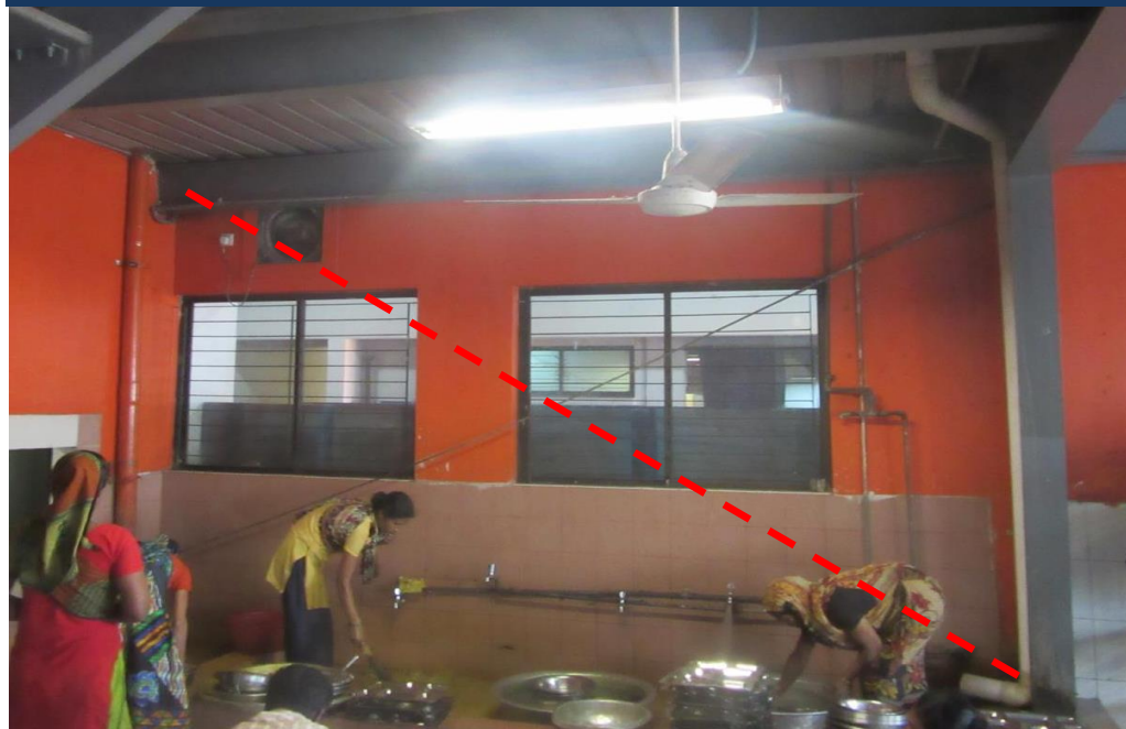
Location of missing vertical bracing.
