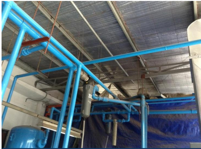
5. Lightweight Roof in Building 4
