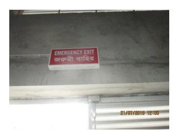
F-18 Egress Lighting Manual on-off switch is provided for emergency lighting and exit signage units. Remove manual on/off switches from emergency Lighting & exit signage units to prevent them from being switched off.
