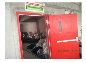
F-4 Fire Rated Construction Unsealed electrical shaft is located in the fire-rated floor/ceiling assemblies. Provide a minimum 2-hr firerated shaft to separate the utility risers from each floor level and seal all penetrations in floor/ceiling assemblies to maintain the fire separation. Within 3 months
