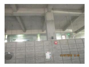
F-8 Fire Rated Construction Exterior exit stair is not properly separated the building interior.
