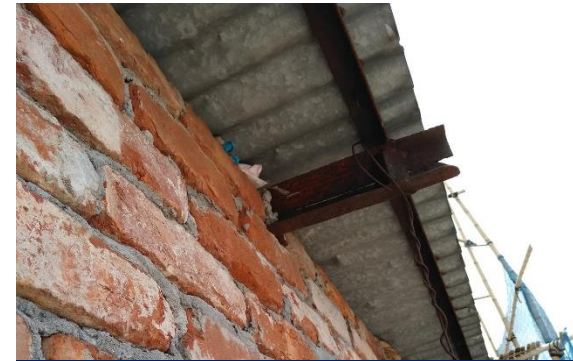
Non-engineered connection
