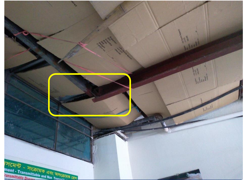
Poor/non-engineered connection was found at extension of shed-1 (doctor's room)
