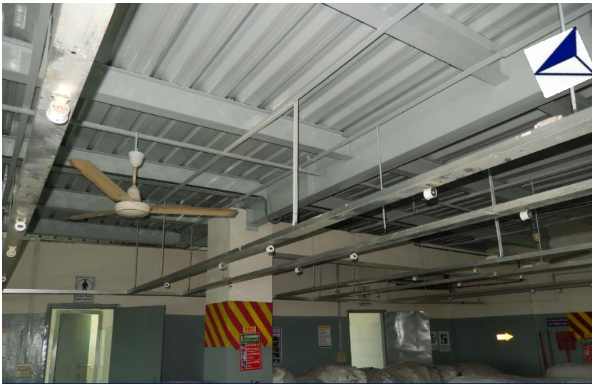
As-built: Primary N-S, purlins E-W direction
