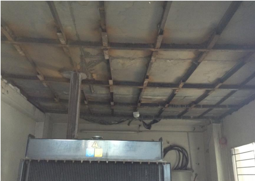
Metal sheet with concrete fill in generator building
