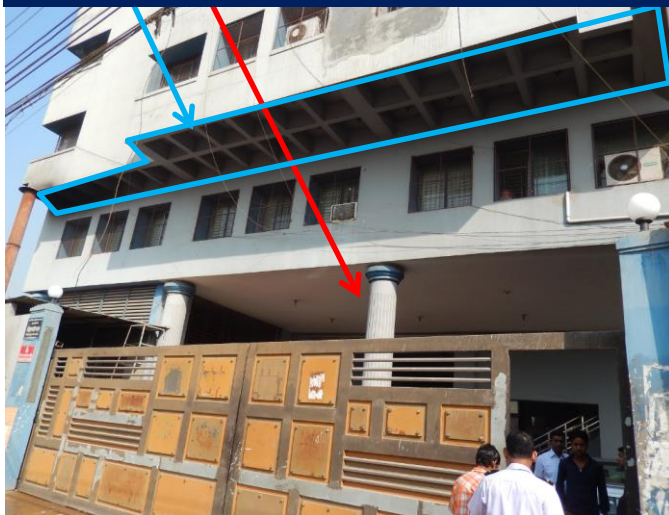
Column supporting cantilever
