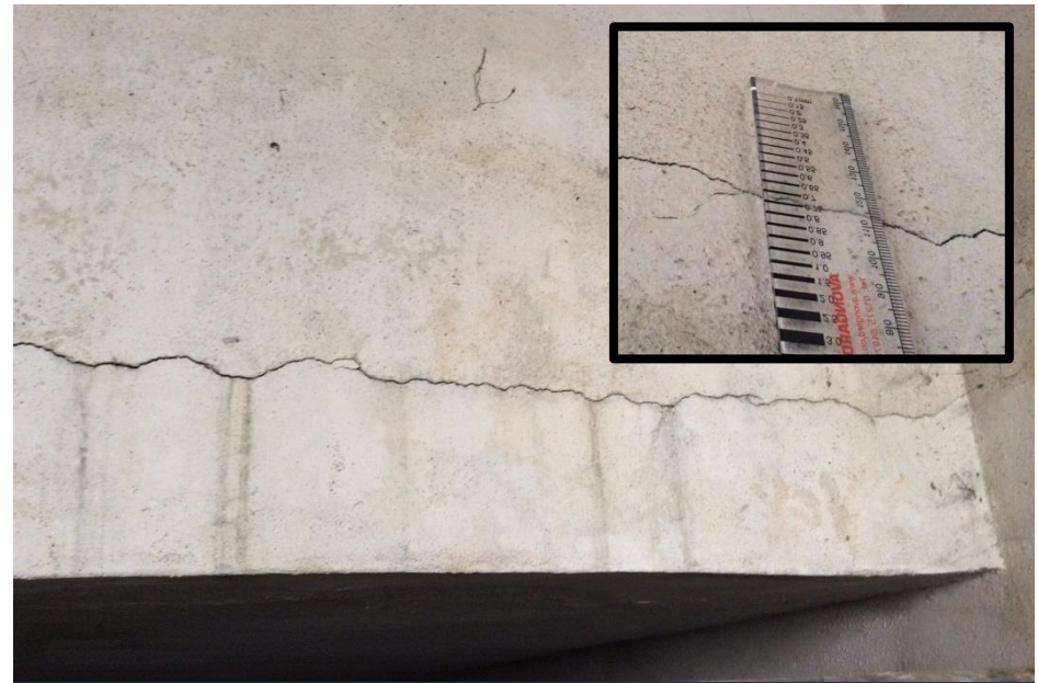
Water Tank Structure
