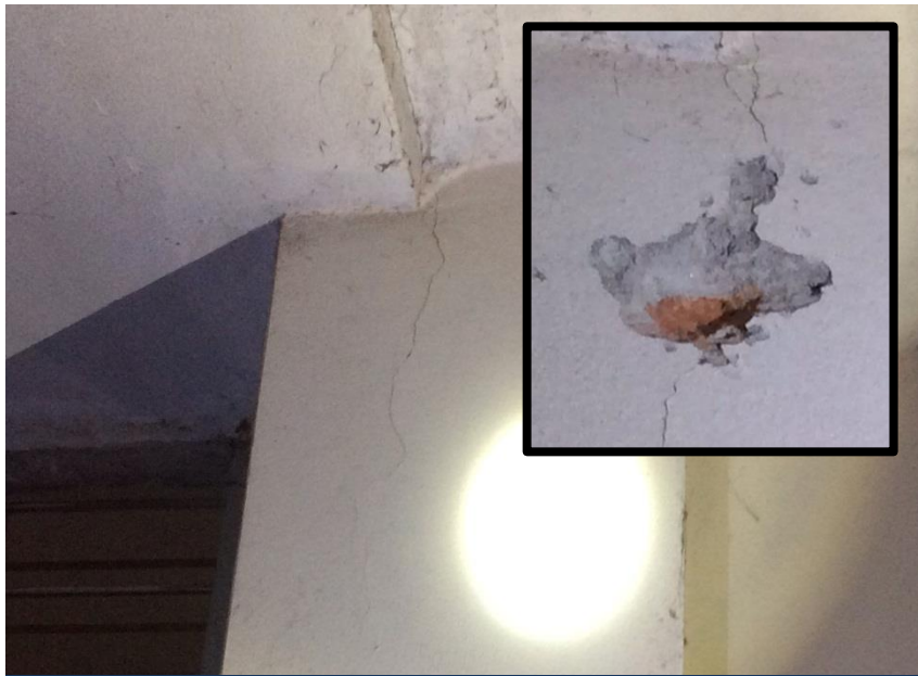
Brick Column at Ground Floor
