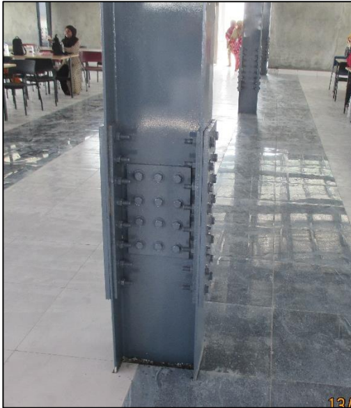
Column Splice in roof
