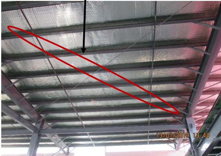
Roof bracing in between grid 5 to 7
