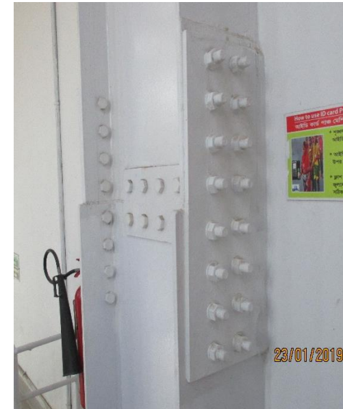
Typical column splice
