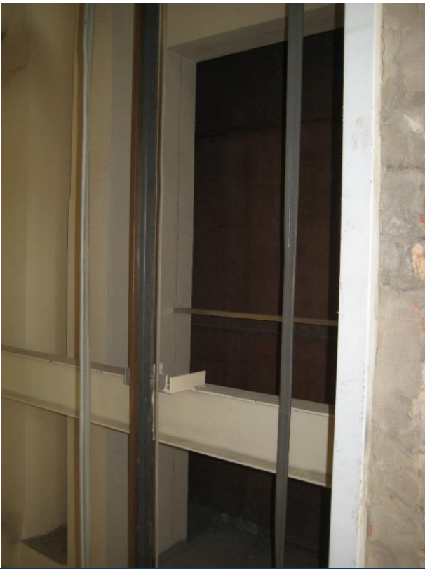
View towards grid 1 from lift shaft G'-G'. Bracing not present
