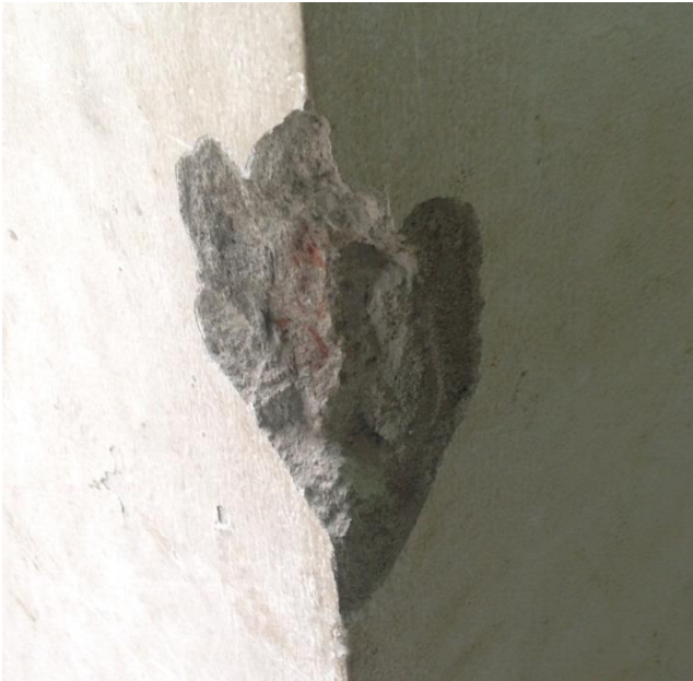
Testing of columns confirmed brick aggregate.
