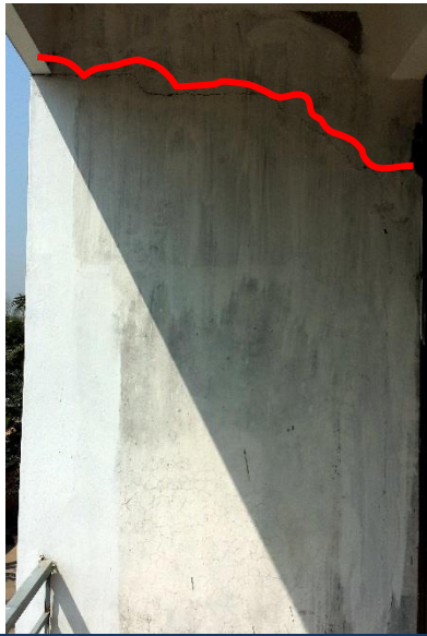
Cracks on the wall in the cantilevers. The cracks width reflects deformations, smaller in bottom , larger at top
