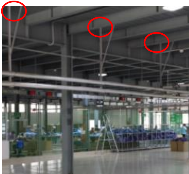
Non-engineered welding of the hanging of the secondary steel work
