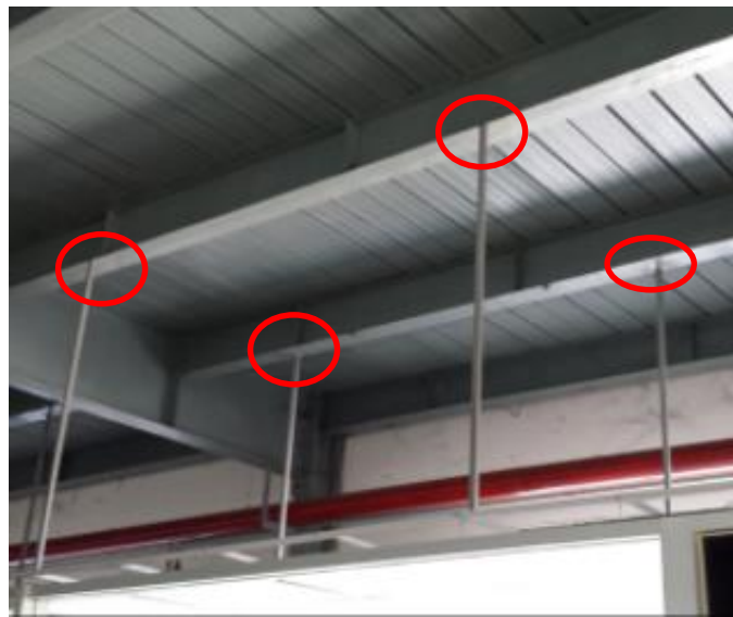
Non-engineered welding of the hanging of the secondary steel work
