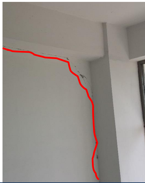
Cracks on the wall in the cantilevers. The cracks width reflects deformations, smaller in bottom , larger at top
