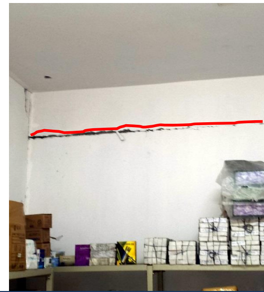
Cracks on the wall in the cantilevers. The cracks width reflects deformations, smaller in bottom , larger at top
