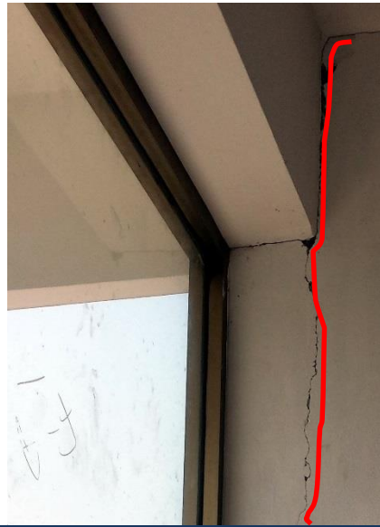
Cracks on the wall in the cantilevers. The cracks width reflects deformations, smaller in bottom , larger at top
