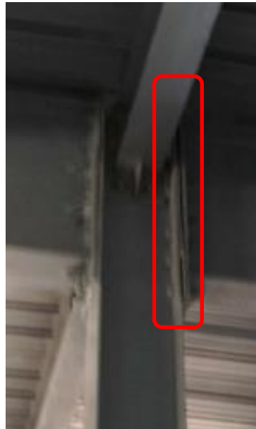
Gaps in the bolted connections in many places, require design check
