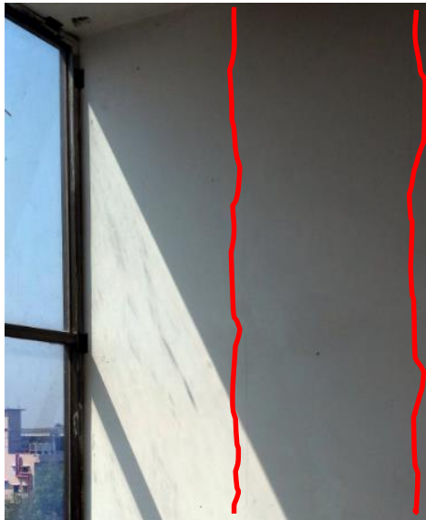
Cracks on the wall in the cantilevers. The cracks width reflects deformations, smaller in bottom , larger at top
