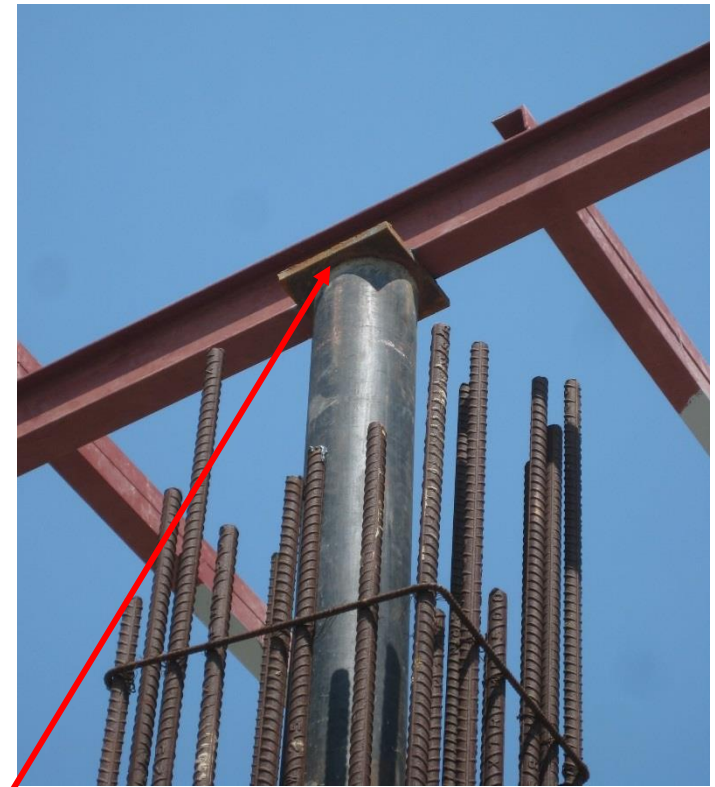
Rafter/post and post/column connection details could not be determined during survey.
