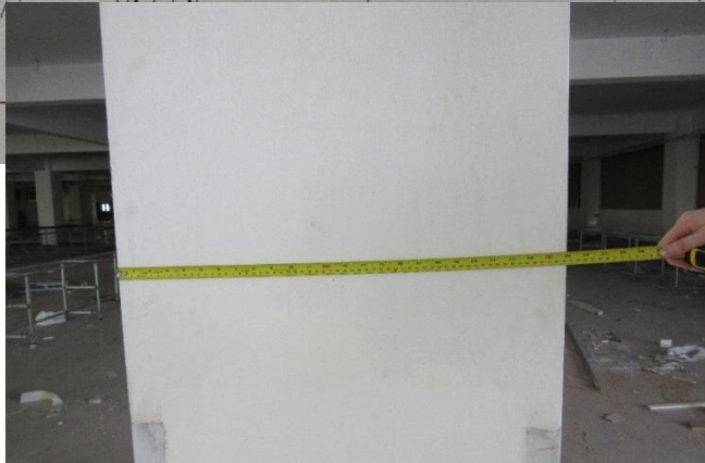
Internal column measured at 5 th floor
