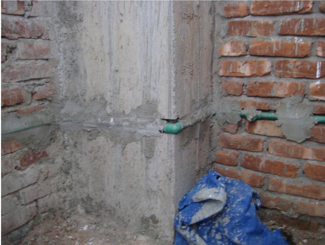
A pipe has been chased into a column at 3 rd floor in the office building
