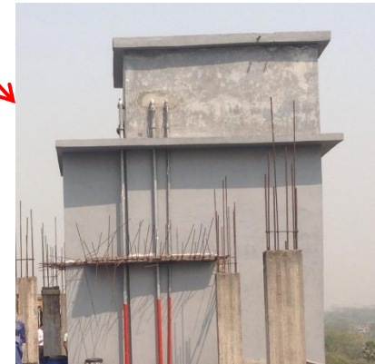
Stair Core & Water Tank
