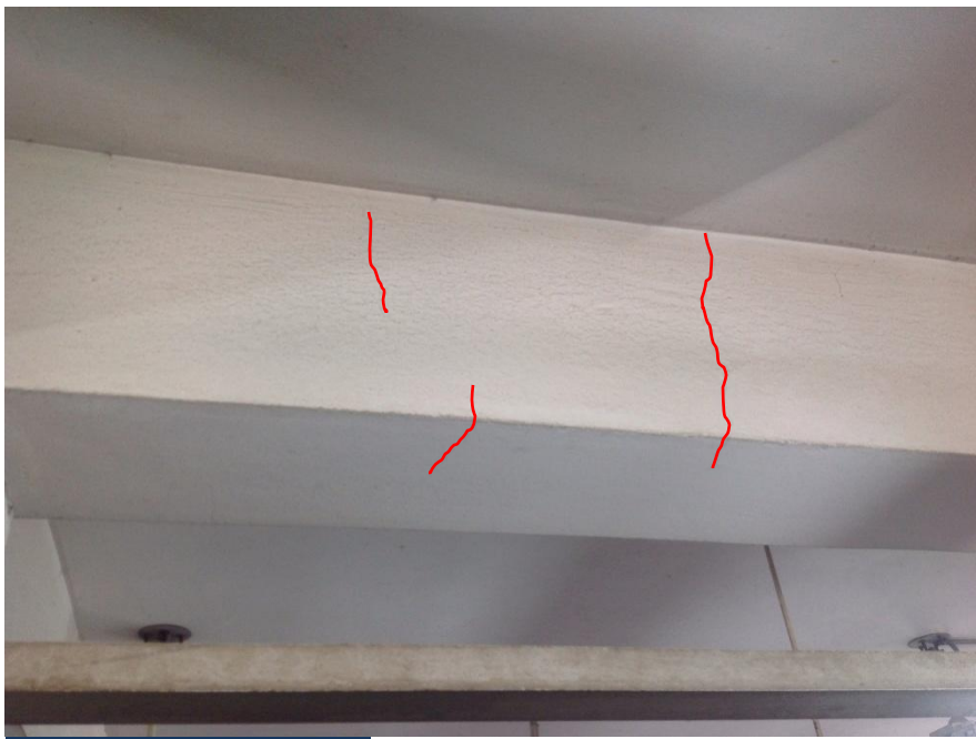
Beam Cracking
