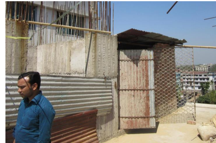
Roof above stair core at front of building
