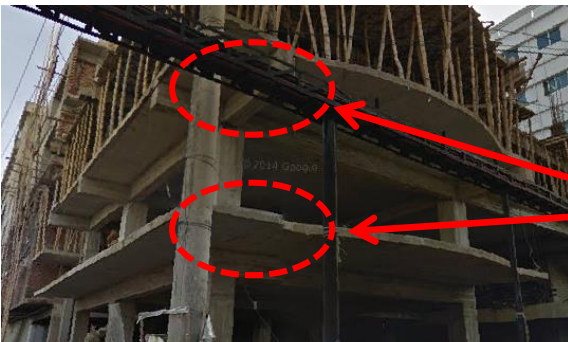
Construction photo of front cantilever (Google)
