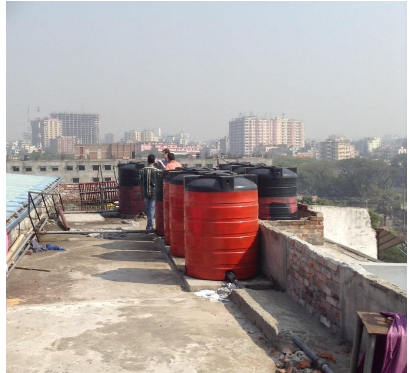
Water tanks on roof over west stair
