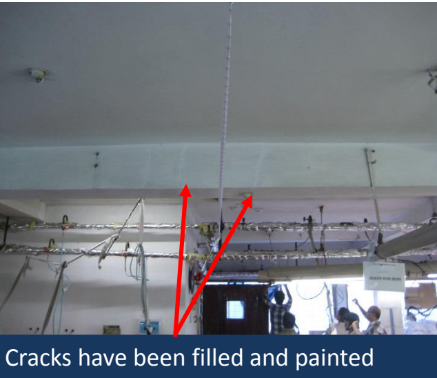
Beam cracking
