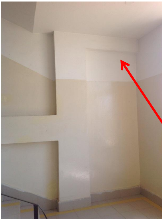
Stairwell cantilever beam
