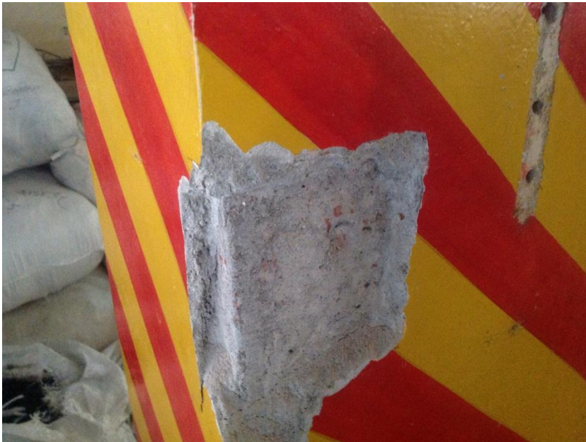
Tested Ground Floor Column – Brick Chip aggregate concrete
