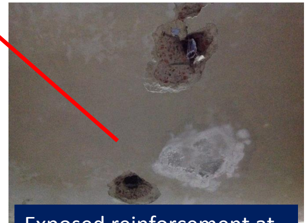
Exposed reinforcement at soffit to beam supporting roof slab in Building 2.
