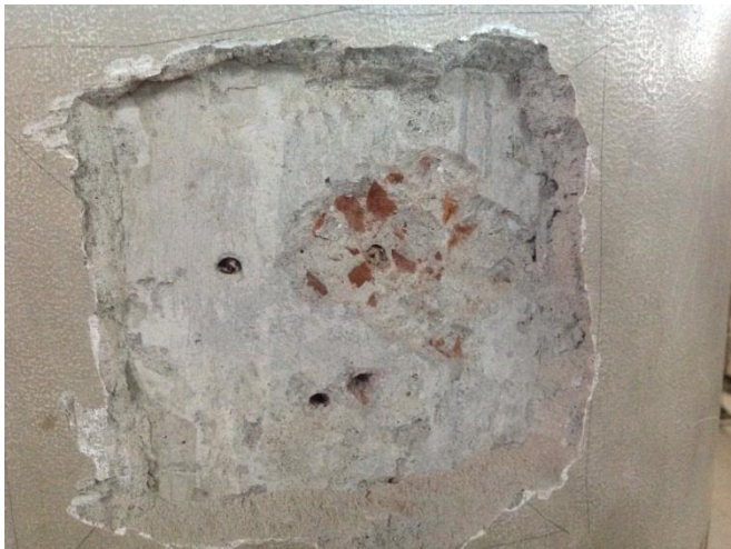
Tested Ground Floor Column – Brick Chips
