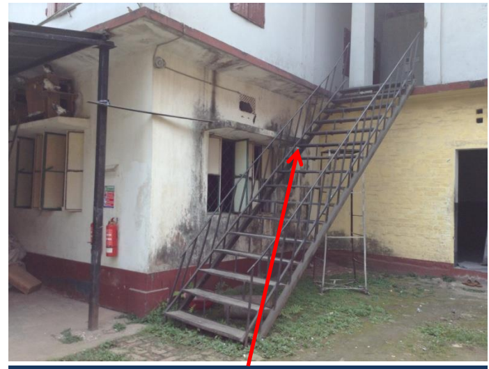
Stair is constructed from small structural sections
