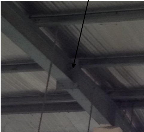
Missing Connection bolts
