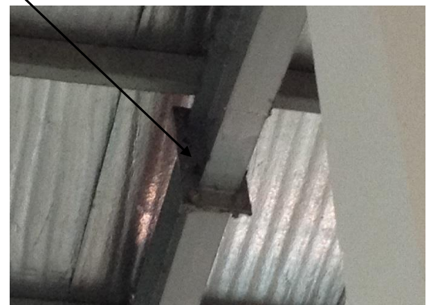
Missing Connection bolts
