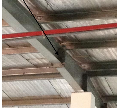
Missing Connection bolts
