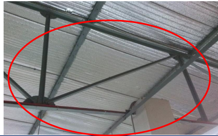
The sizes of structural members are very small (L-shapes L50 x 5 to L70 x 7)
