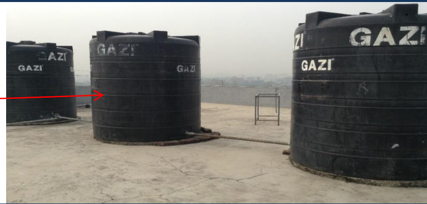
3 Water tanks on roof – 5000 litres each (total 1500 kN)
