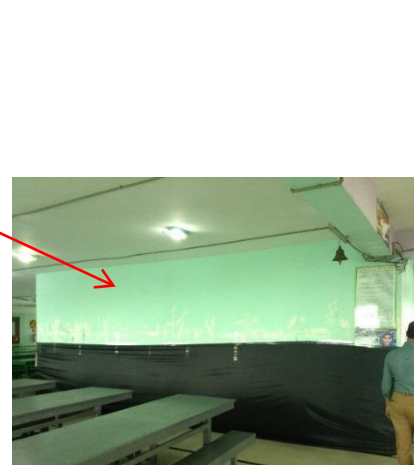
Water tank on 8 th floor
