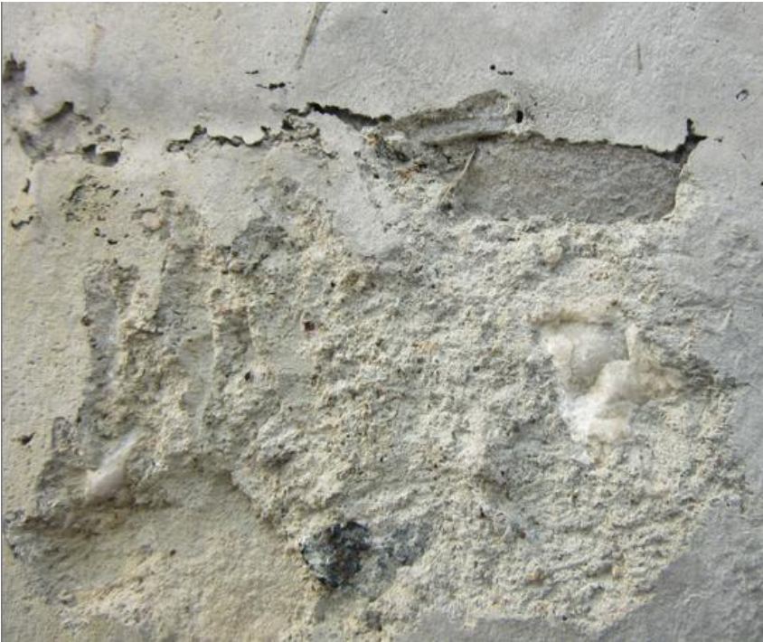
Stone aggregate in the Main Production Building B1
