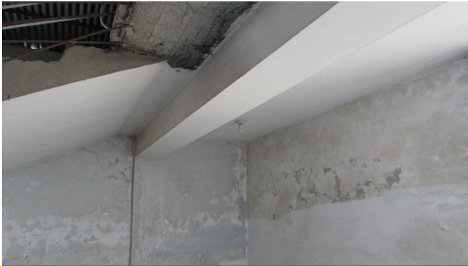
Water ingress on the stair wall
