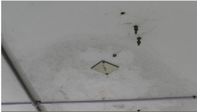
Cracks and water ingress on the ceiling of 4 th floor level
