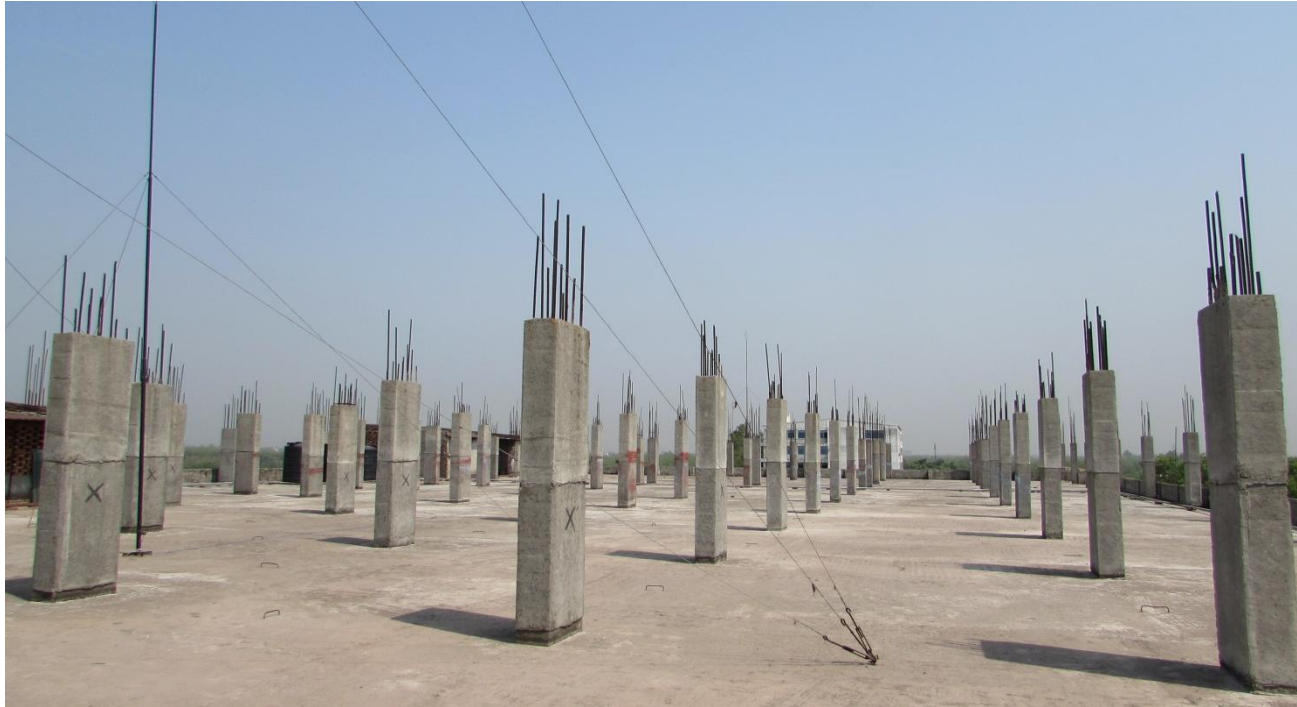
Lack of proper waterproof layer
