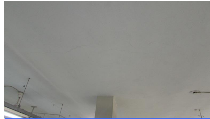
Cracks on the soffit of lower levels.
