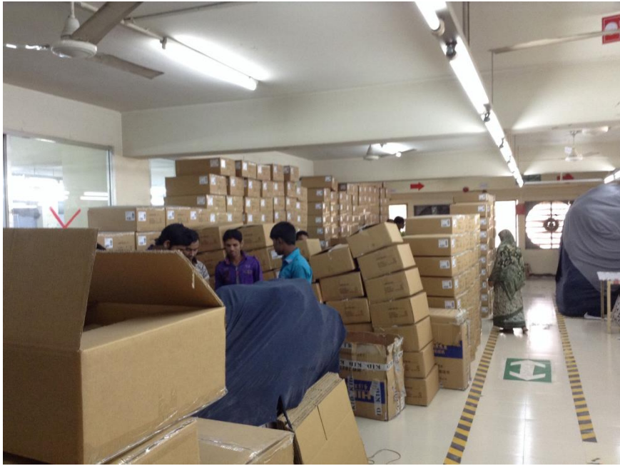
Heavy loads, approximately 5kPa to 8kPa observed on 1 st floor
