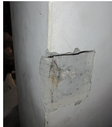
Stone Aggregate (Ground Floor)
