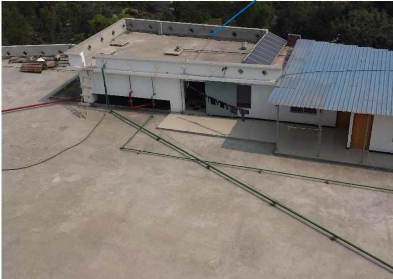
RC water tank (43000L) on 6 th floor roof
