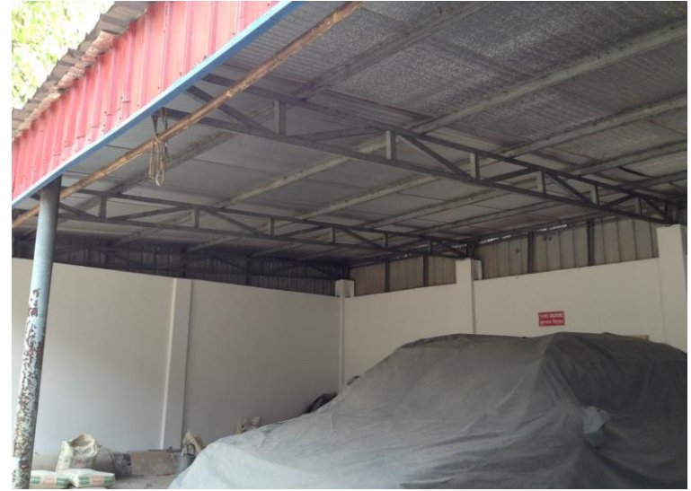
Non engineered roof structure to garage
