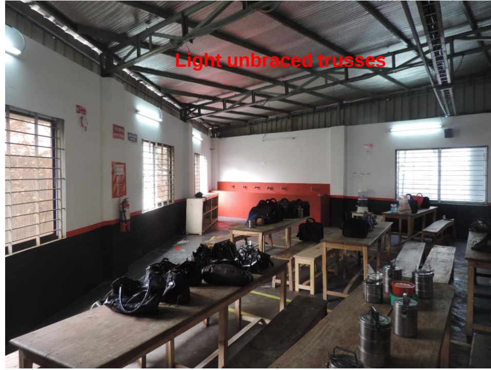
Non engineered roof structure to Dining and generator building 5
