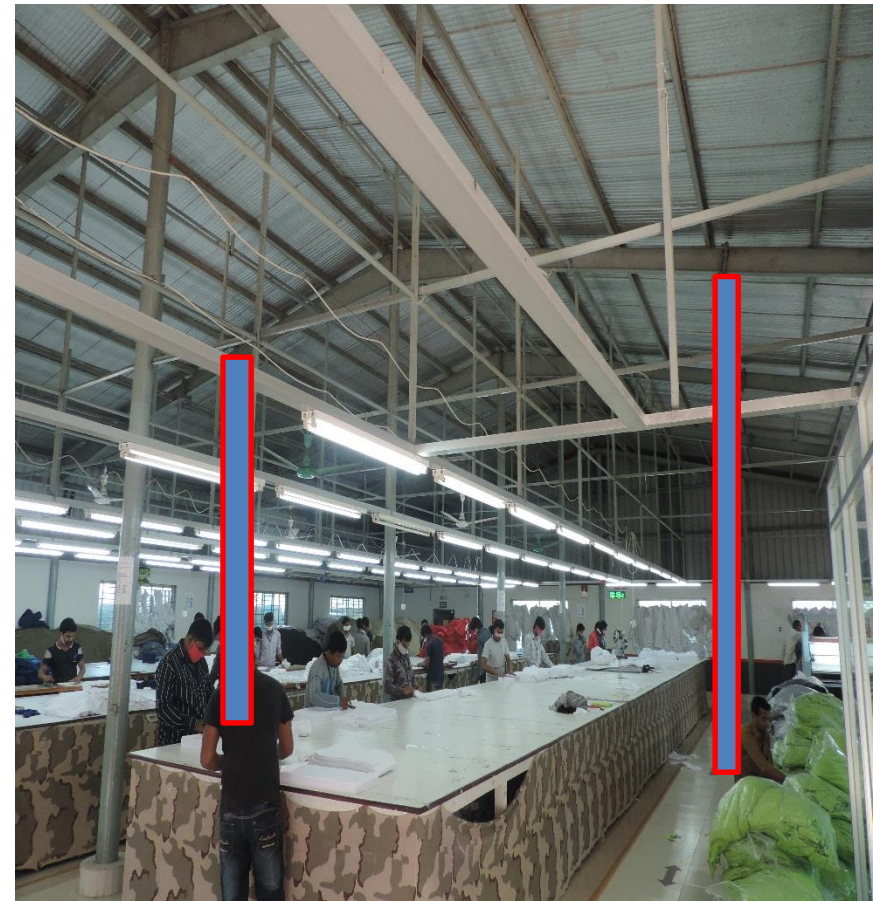
No column was found during inspection
