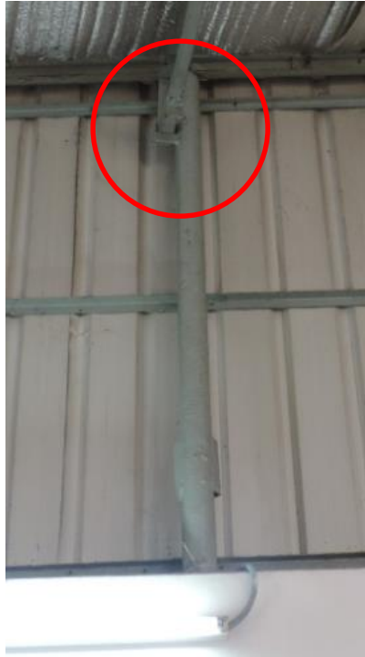
Non engineered roof structure to Dining and generator building 5
