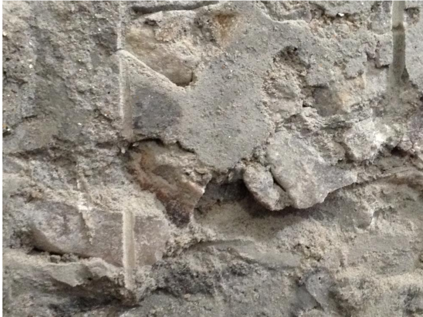
Stone aggregate in Building 1
