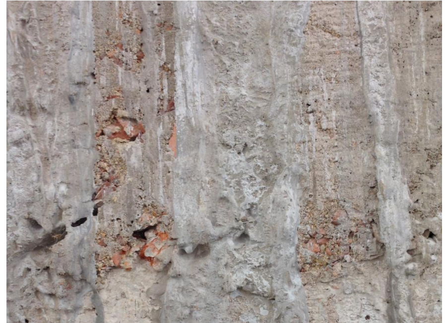
Brick aggregate present in the Buildings No2 & No 3
