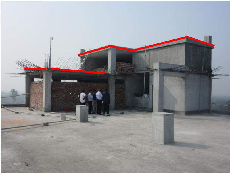
No edge protection was provided on the roof (marked with red line)
