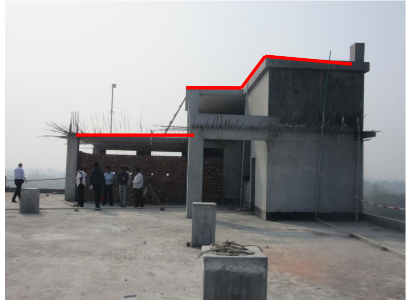
No edge protection was provided on the roof (marked with red line)
