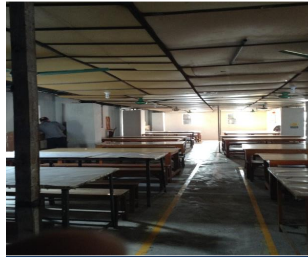
Non-engineered structure at roof top
