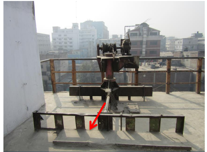
Hoist on the front side of the roof
