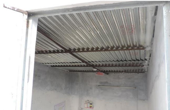
Non-engineered structure over the stair core
