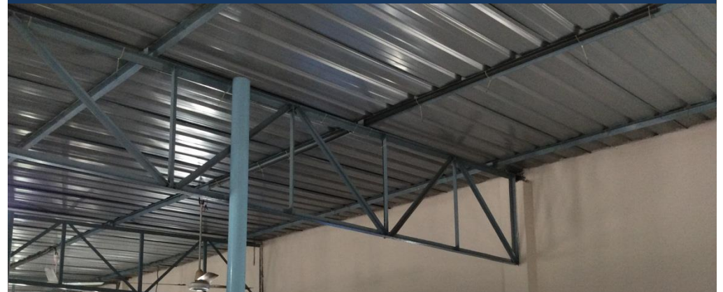
Dining/Prayer room – roof truss appeared to be hanging from box section columns
