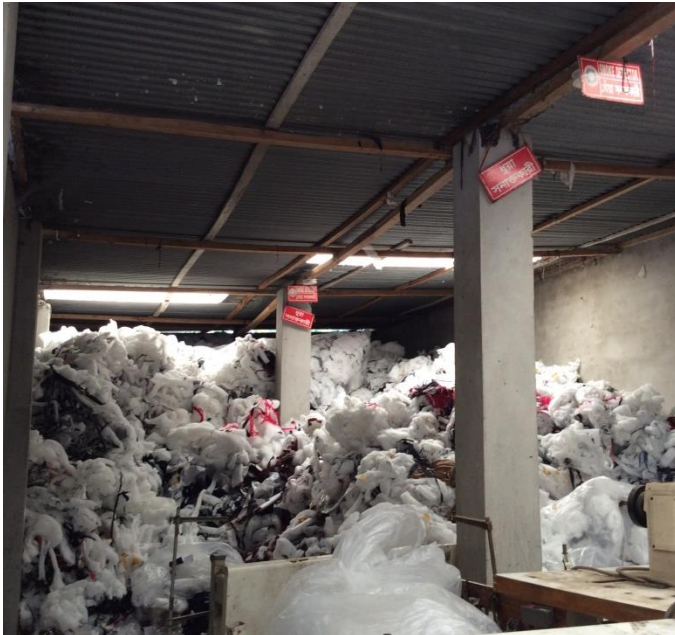
Storage Shed – steel roofing on timber purlins positioned on concrete columns
