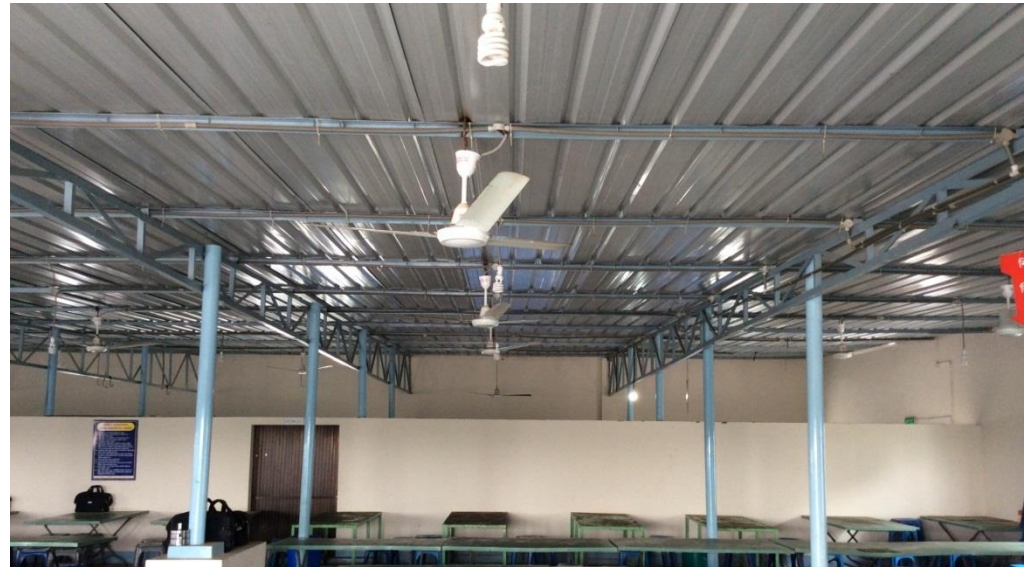
Dining/Prayer room – roof truss appeared to be hanging from box section columns
