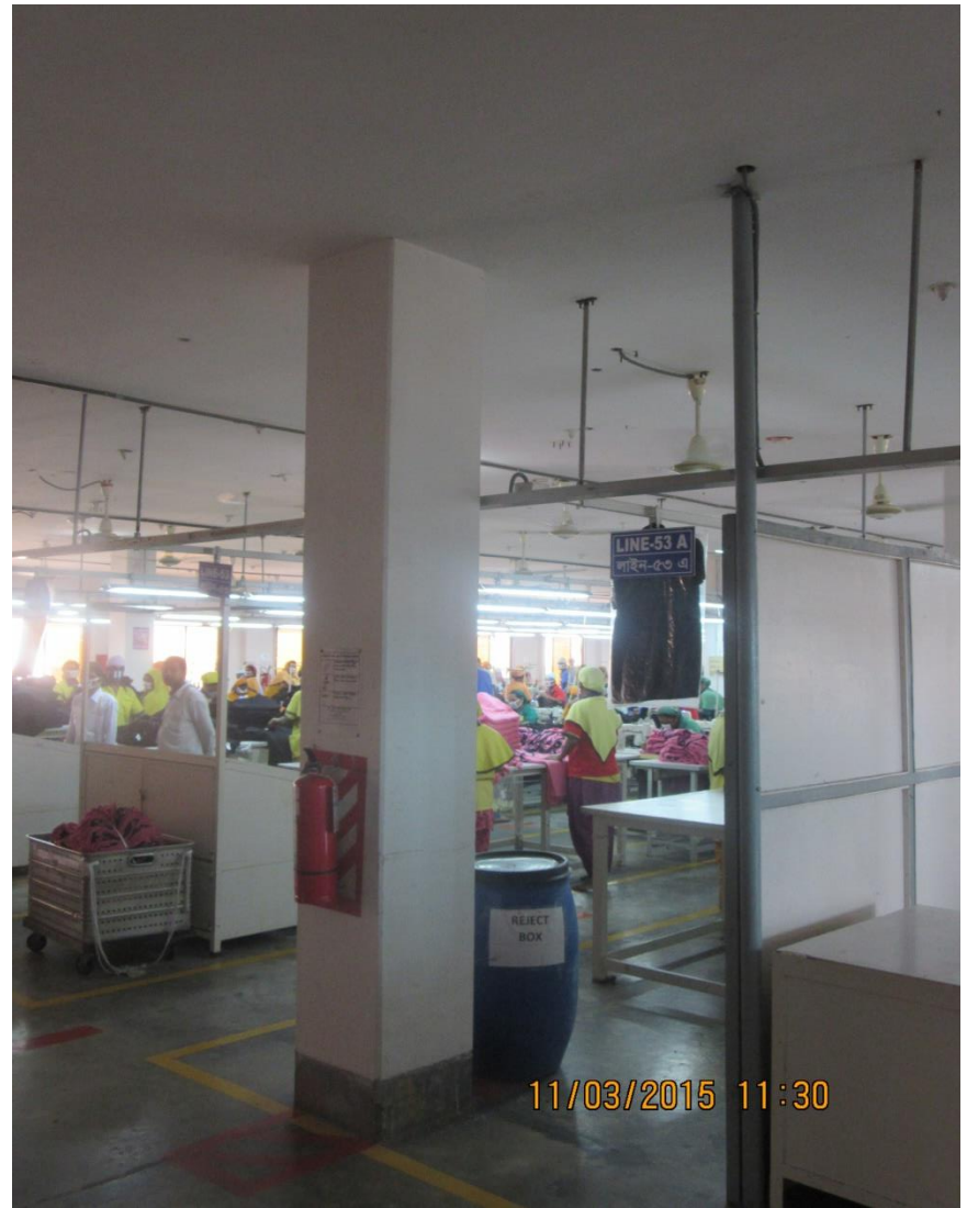
Flat slab from 2 nd floor and above
