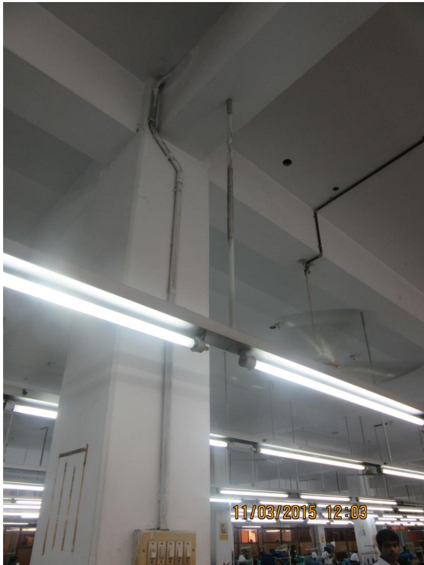
Beams and slab at ground and 1 st floor
