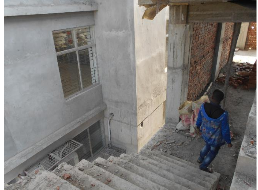
1 st Level near stair
