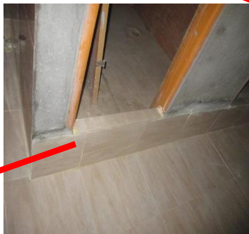
Toilet build up
