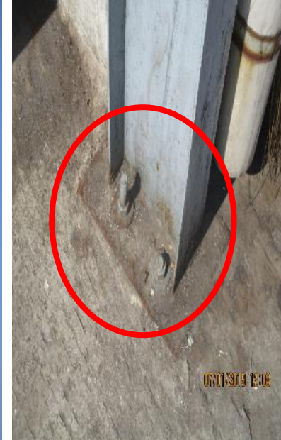
Steel columns were bolted on roof slab
