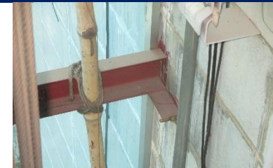
Connection (bolted) between steel frame to building
