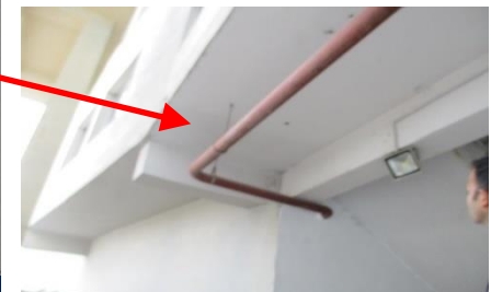
Cantilever at floor level
