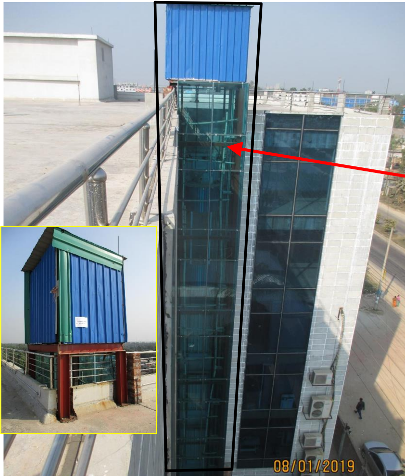
The steel lift core adjacent to main building.
