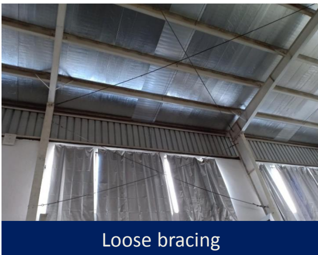
Loose bracing
