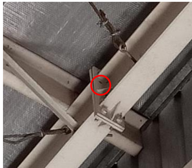
Bolts missing in several location
