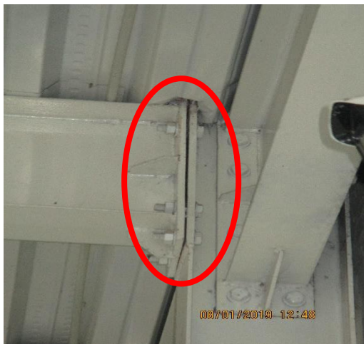
Existence of significant gap at connections
