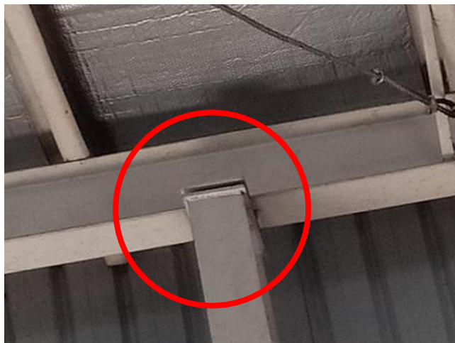
Existence of significant gap at connections
