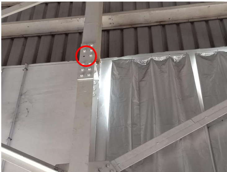
Bolts missing in several location
