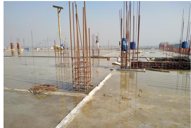
Under construction roof
