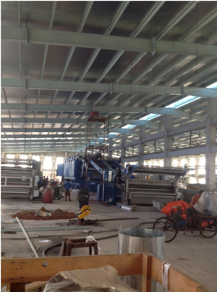
New steel framed warehouse
