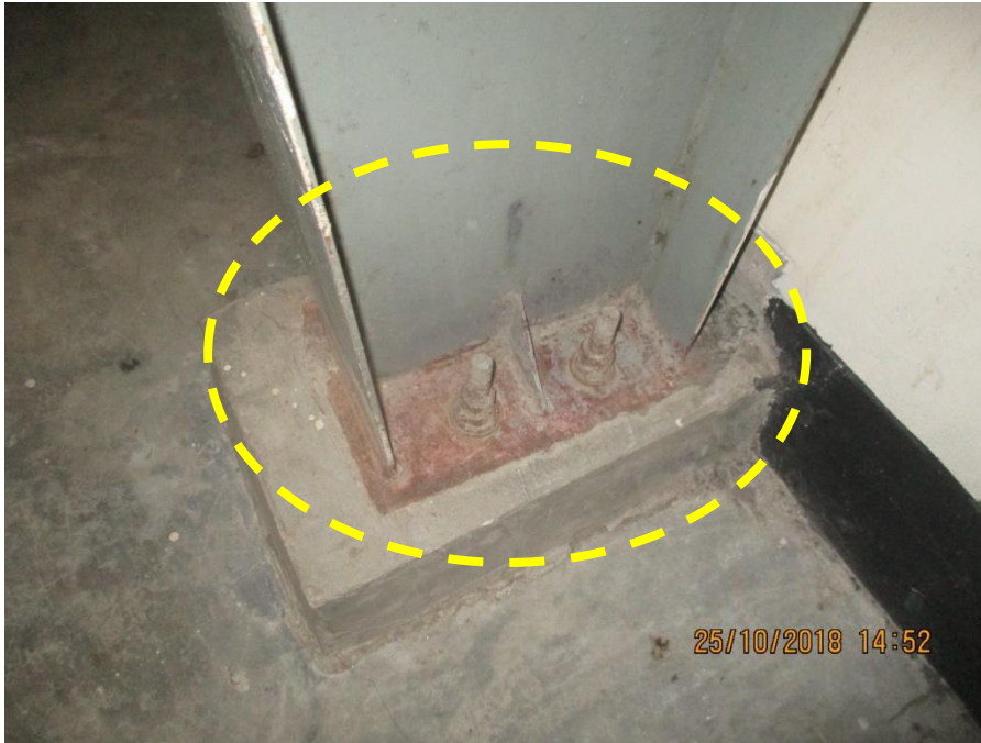
Corrosion was observed at joint of pedestal column and steel column.
