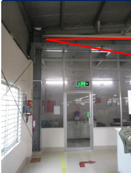
Gap was found in column-beam joint at mezzanine floor
