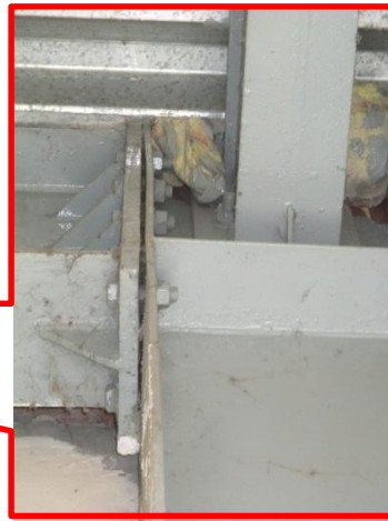
Gap was found in column-beam joint at stair case location
