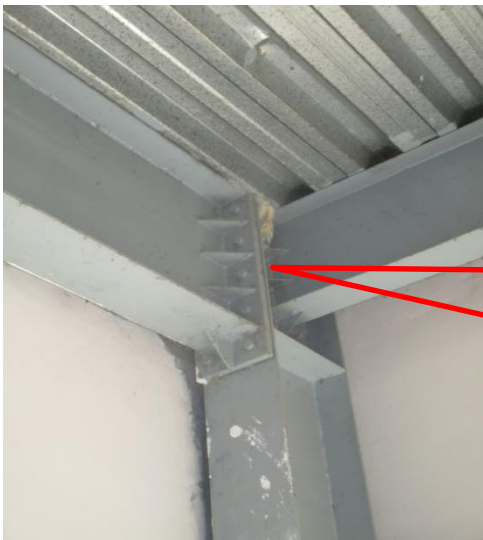
Gap was found in column-beam joint at stair case location
