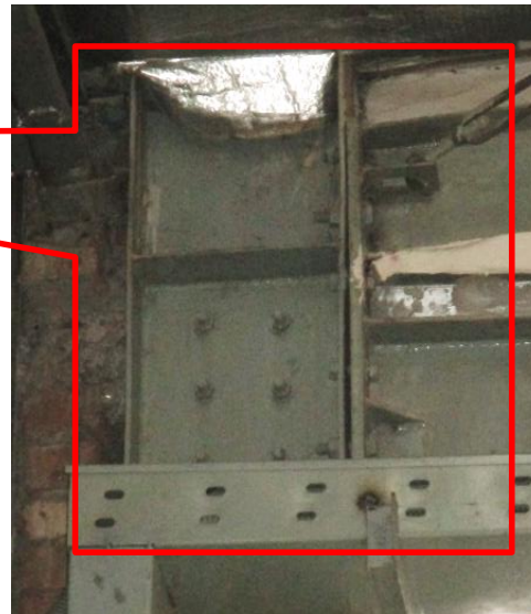
Gap was found in column-beam joint at mezzanine floor
