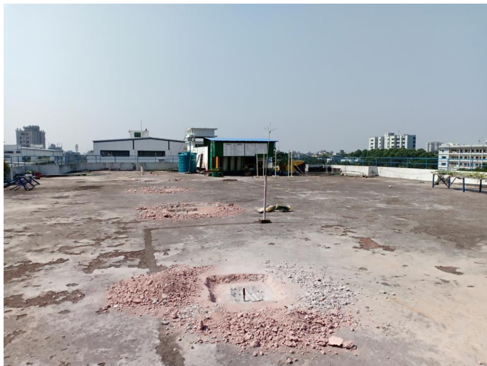
Current roof of factory building
