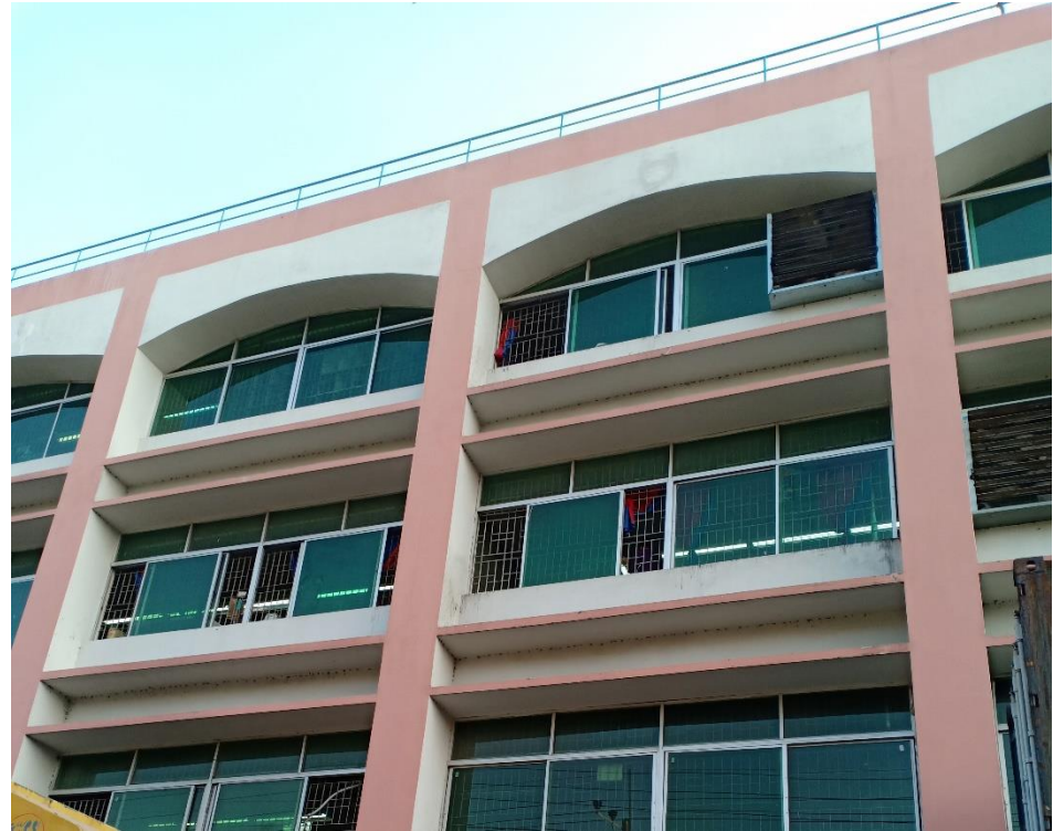
Windows on 2 nd & 3 rd floor
