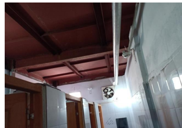
Deck slab at 1 st floor level
