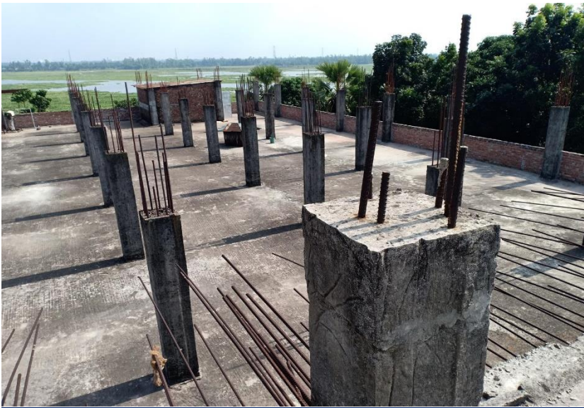
Current roof of factory building
