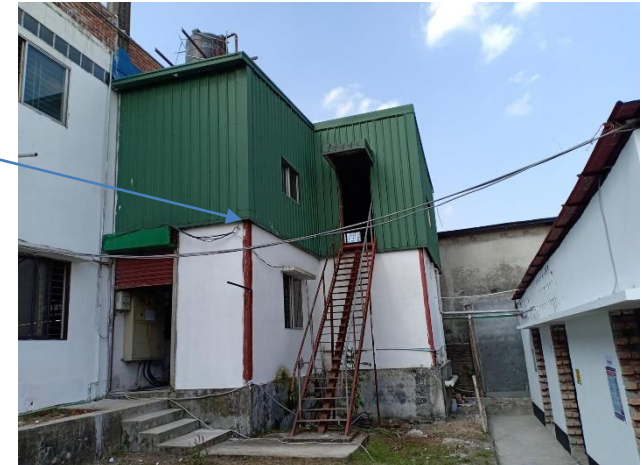
Undocumented steel shed
