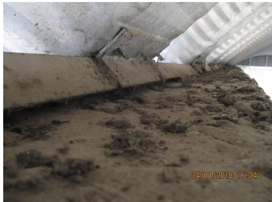
Connection between profiled roofing & support.
