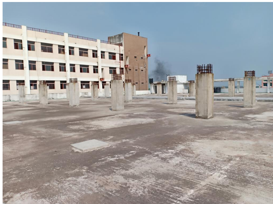
Current roof of factory building
