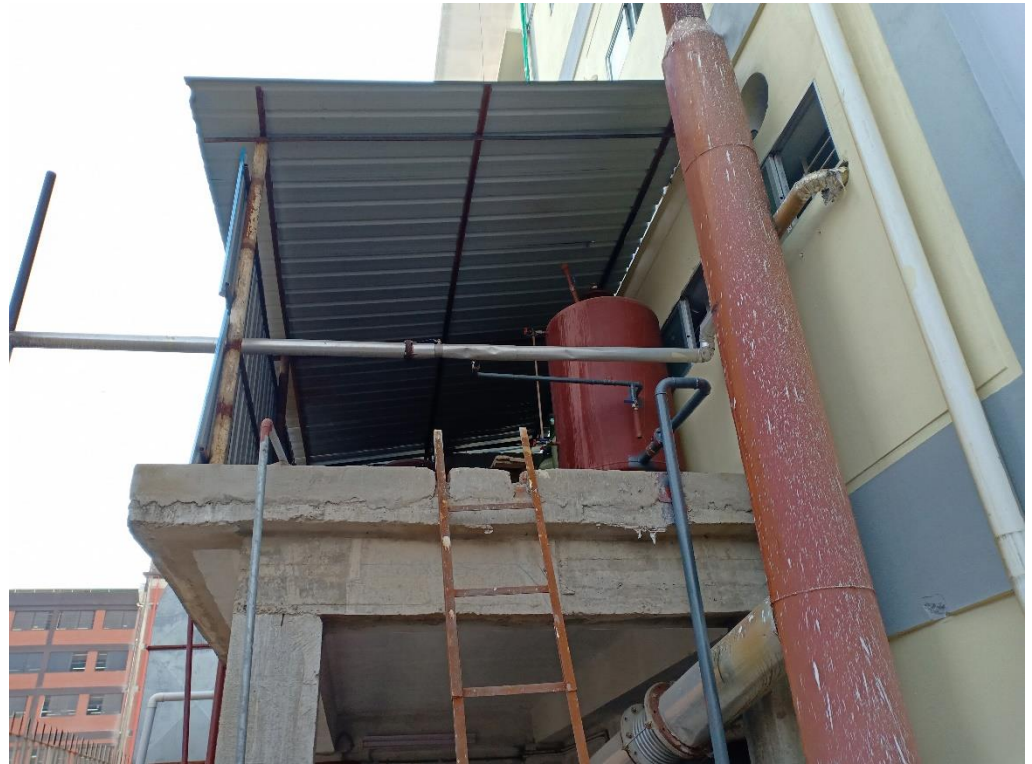
Light weight roof supported by Bamboo
