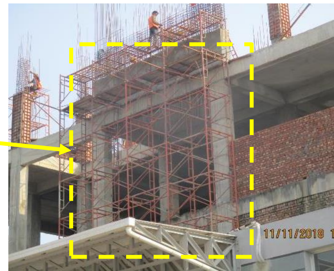
New shear wall construction layout New shear wall is being constructed by top to bottom method
