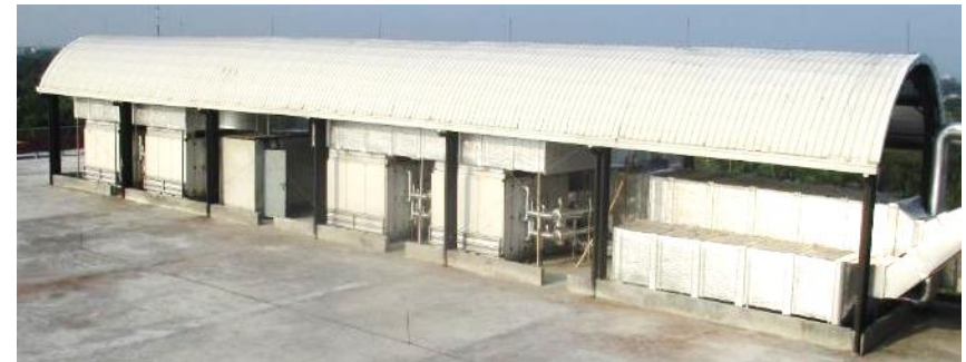
On site location of vertical bracing
