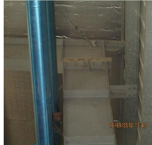
Bolted connection between rafter and column
