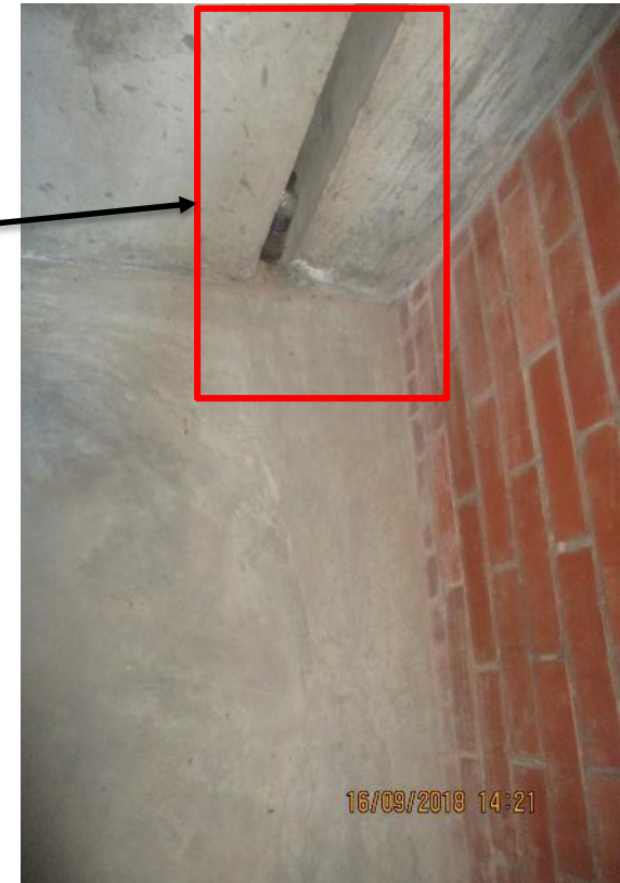
Expansion joint covered with mortar
