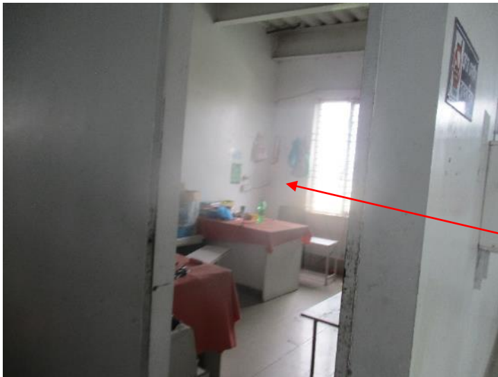
Vertical Bracing missing
