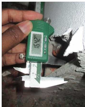
Column thickness 16 mm instead of 20 mm
