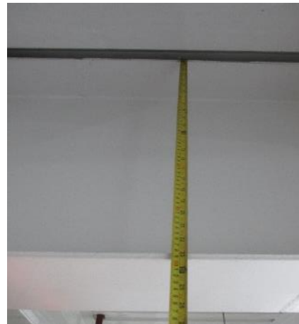
10 mm thickness of flange instead of 12 mm
