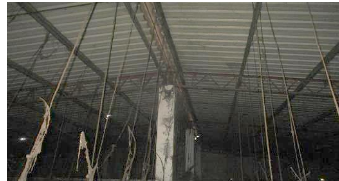
Typical internal truss frame (Field Condition)
