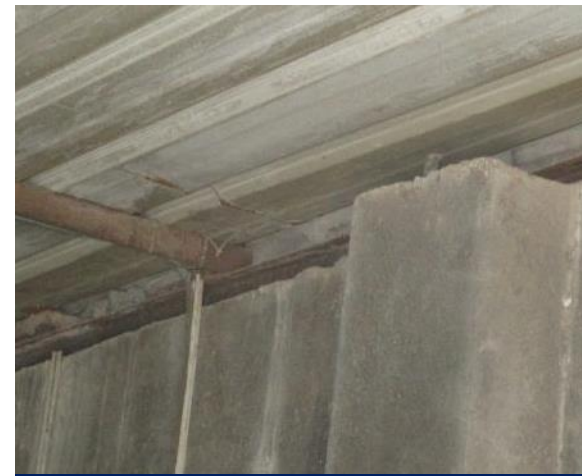
Steel angle was supported on brick wall
