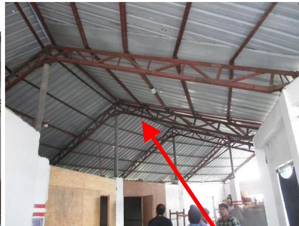
Truss on 3 rd floor
