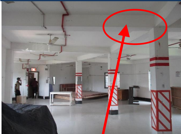
Beam missing in 1 st & 2 nd floor
