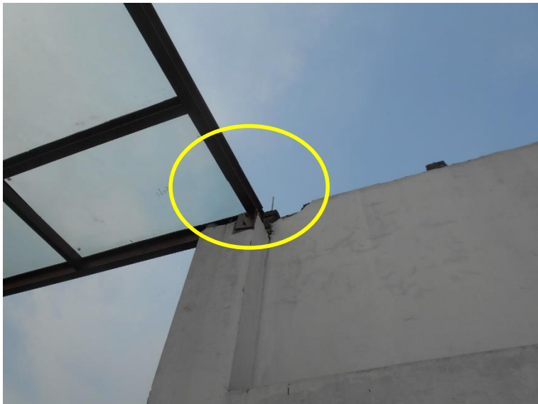
Apparently non-engineered connection was observed in the truss at roof
