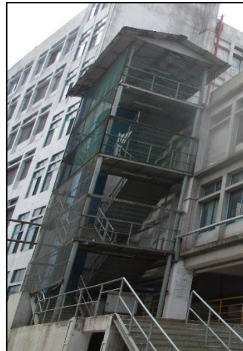
Emergency Steel stair on south face.
