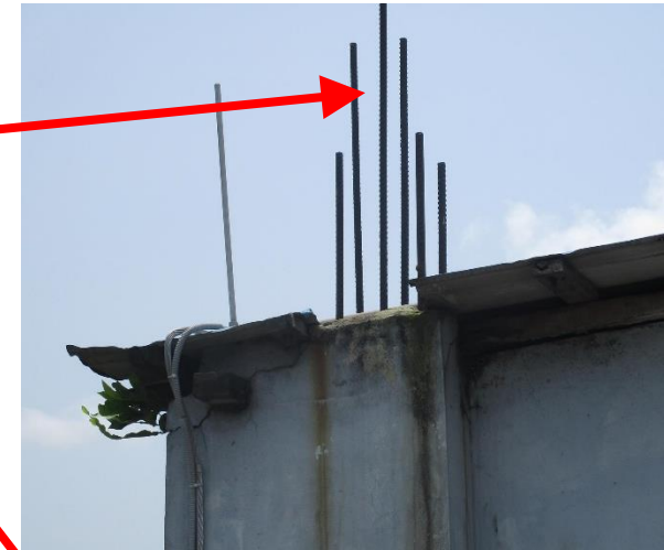
6 Rebars in stair column
