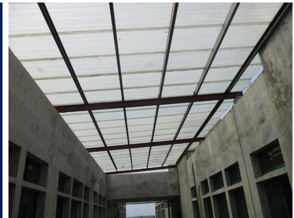
Steel Roof frame of Twin Tower-1 & 2
