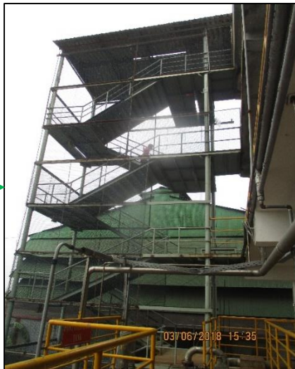
Emergency Steel stair on north face.
