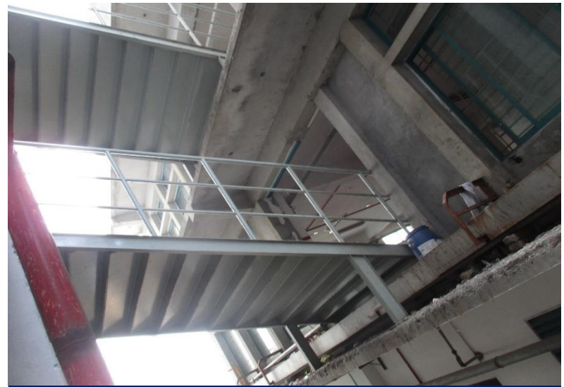
Steel stair in between Twin Tower-2 to ETP
