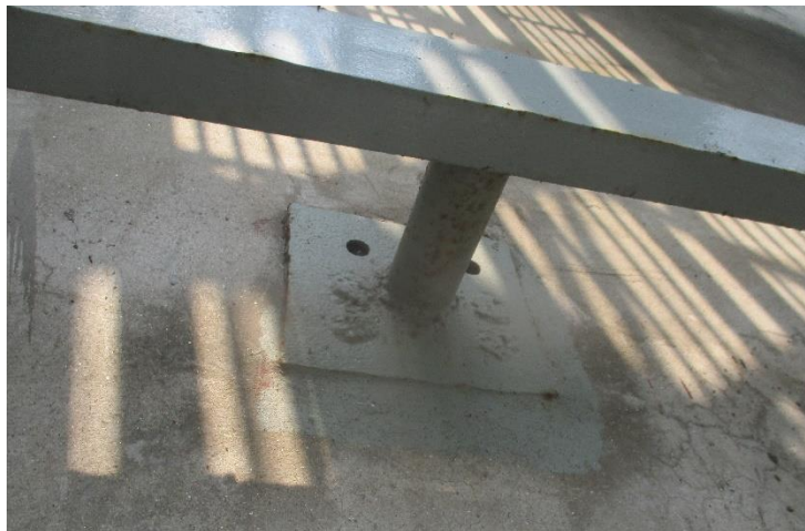
Poor connection
