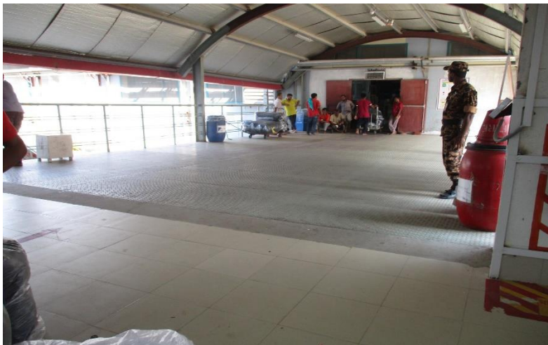
Steel connecting bridge from Twin Tower
