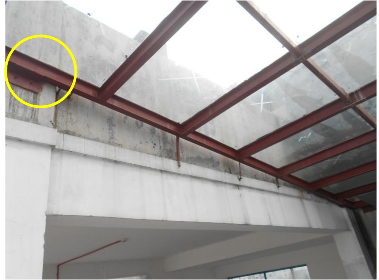
Apparently non-engineered connection was observed in the truss at roof
