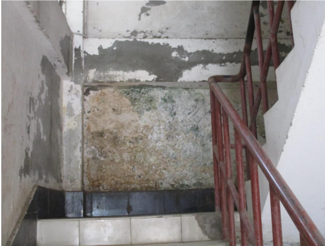
Dampness due to water intrusions was observed in various locations.
