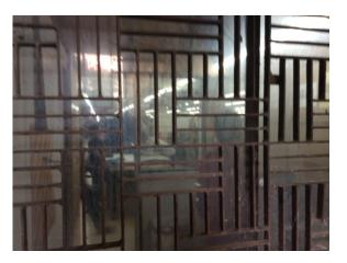
F-2 Fire Rated Construction Areas used for combustible storage are not separated by firerated construction.
