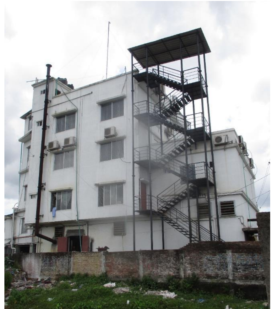
External steel stair at south. No drawing was available during inspection.
