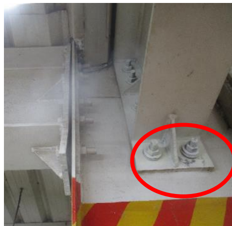
Improper bolt connection
