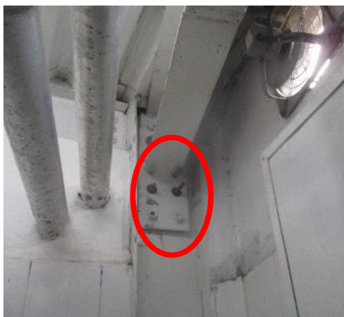
Improper bolt connection
