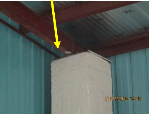
Internal portal frame without any bracing system
