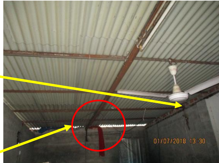
Internal frame of shed
