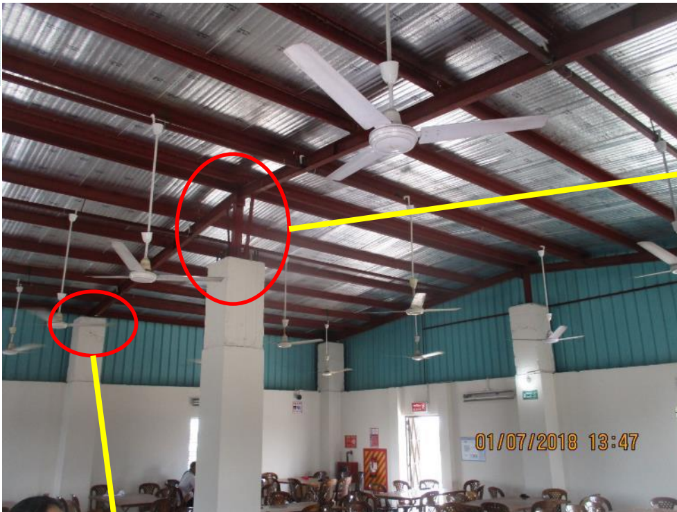
Internal portal frame without any bracing system
