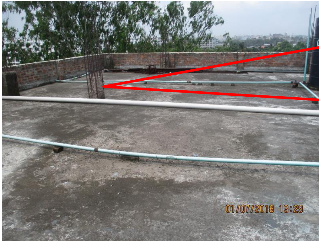
Corrosion was observed on all exposed reinforcement on roof top
